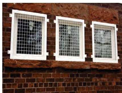
window with wire-netting
